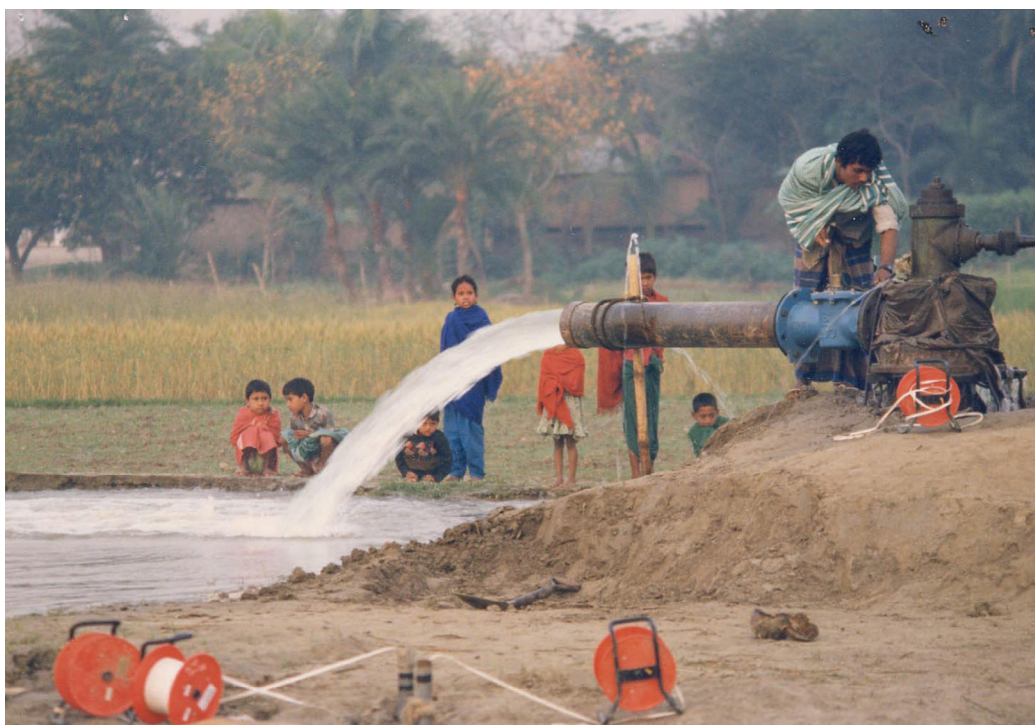
FIGURE 6: A borehole in Bangladesh yielding about 80 L/s
