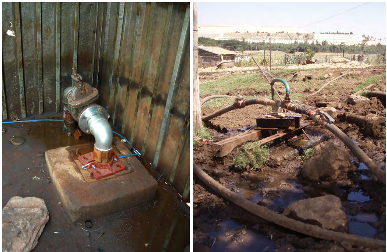
FIGURE 23: Borehole head works contaminated by diesel fuel (left) and agricultural runoff (right)
