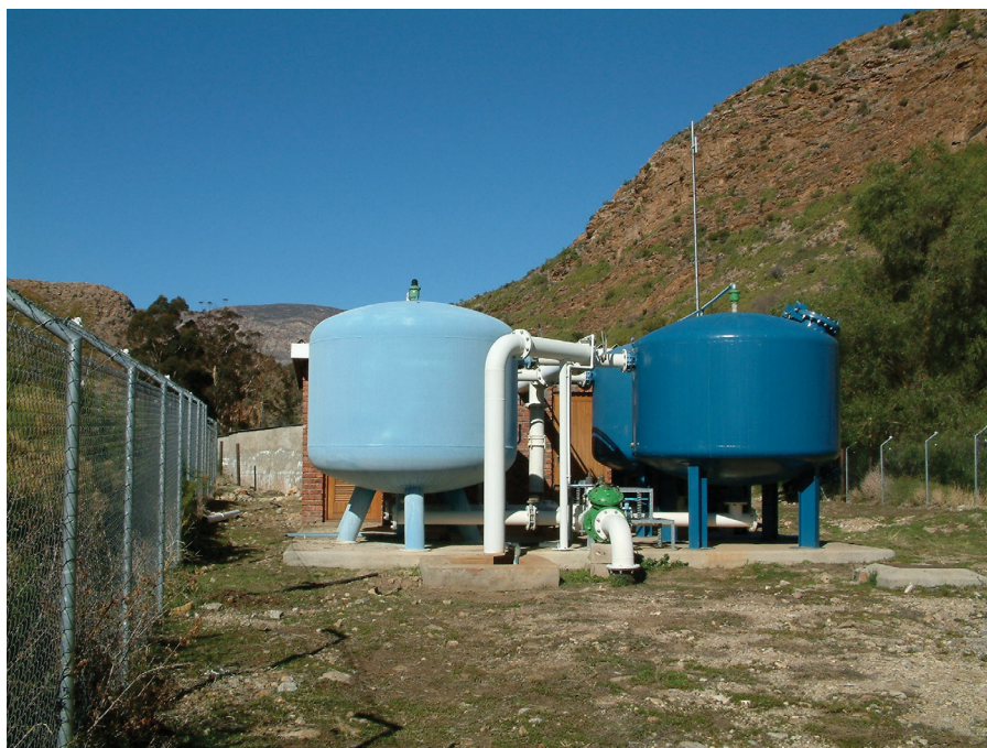
FIGURE 11: Sand filters (treatment step 3) at a small town water supply in South Africa
