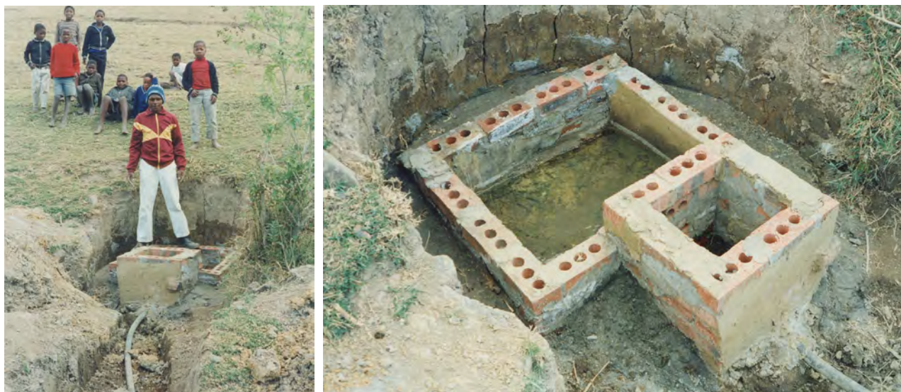
FIGURE 15: A spring protection being installed in South Africa
